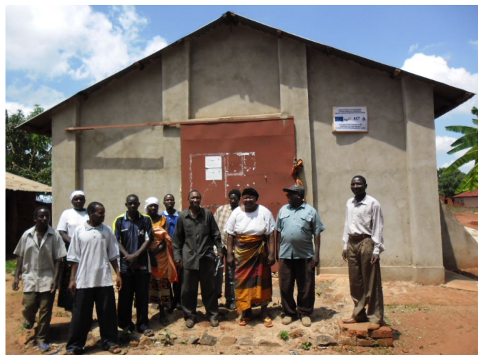
Figure 7: Mngazini Warehouse - Upper Photo - Front View, Lower Photo - Rear View
